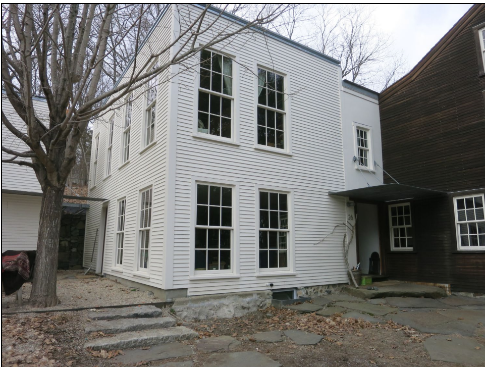
Former attached barn renovated for kitchen on first floor.
