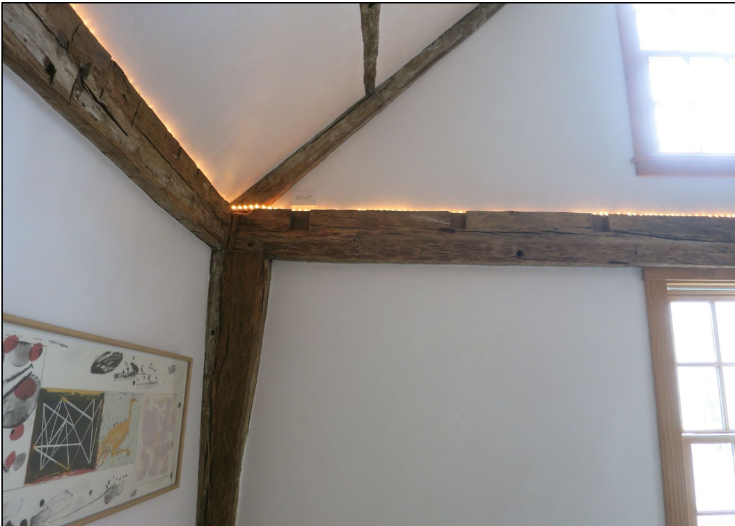
Second floor, SE corner showing gunstock post, girts, rafter and purlin.
