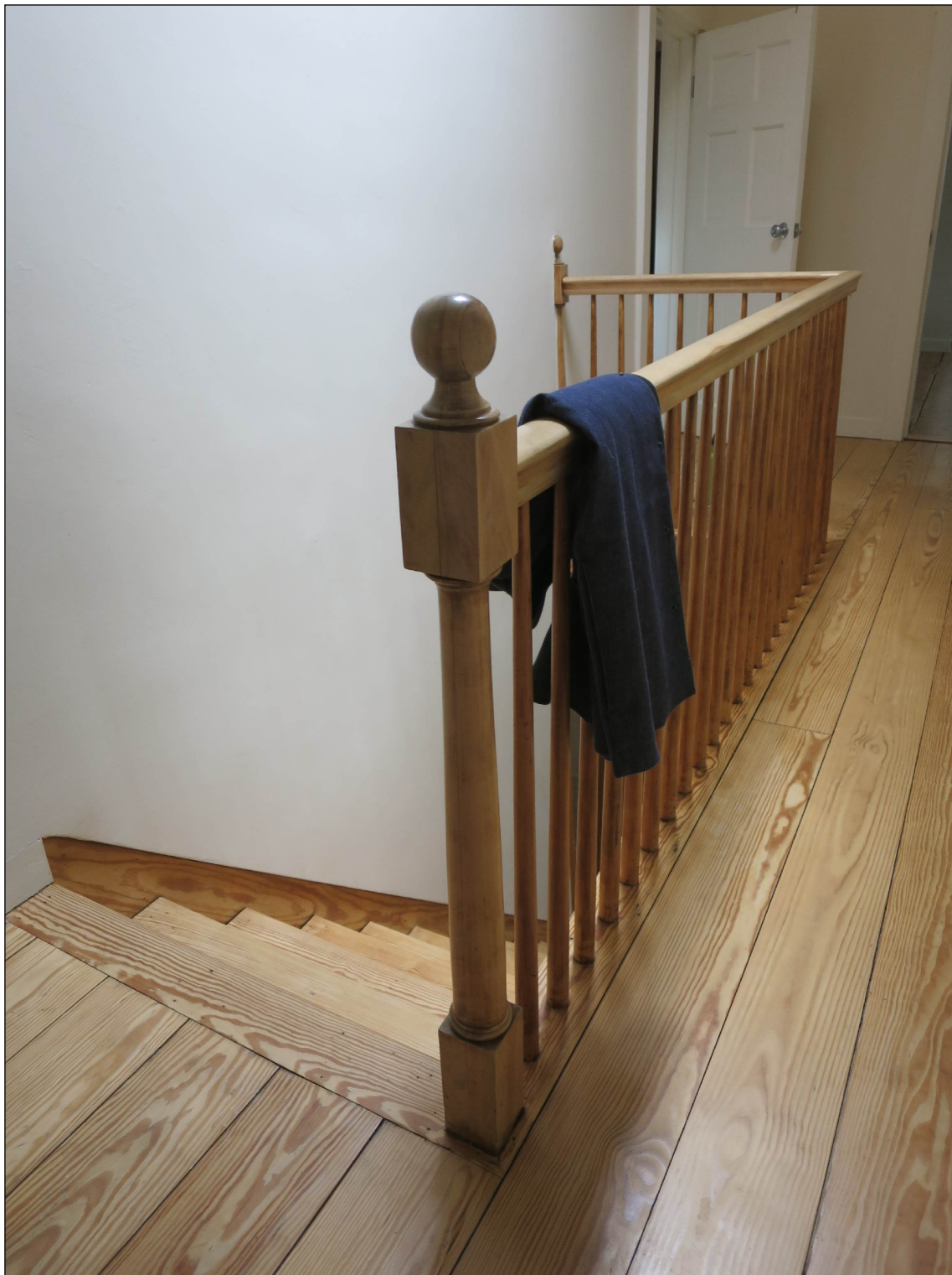
New stair in lean-to.
