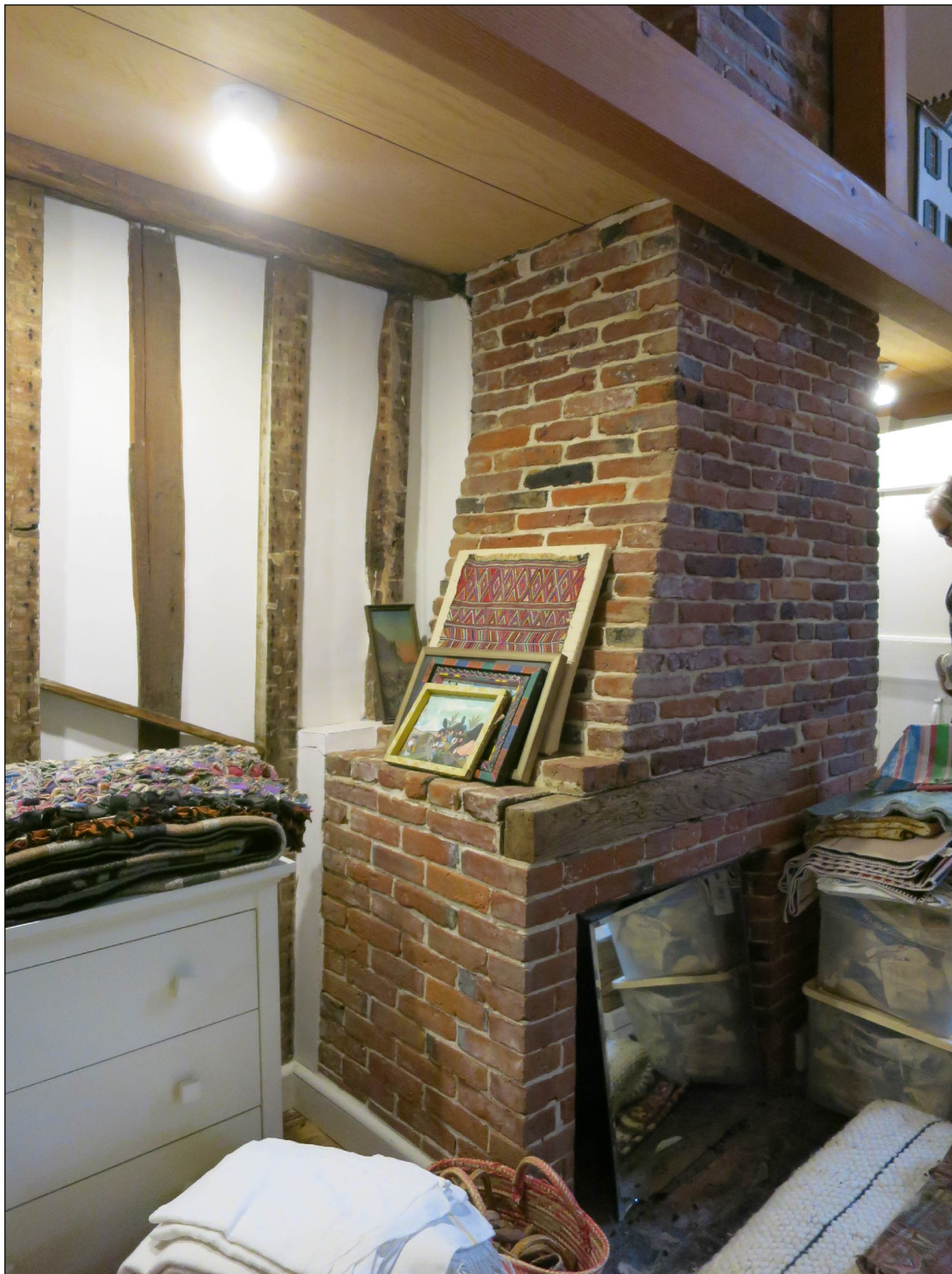
Second floor fireplace and chimney showing studs for lean-to partition.
