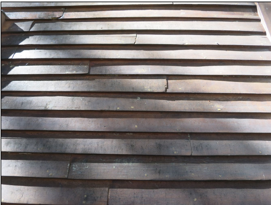
Detail of original clapboards found under vinyl siding.
