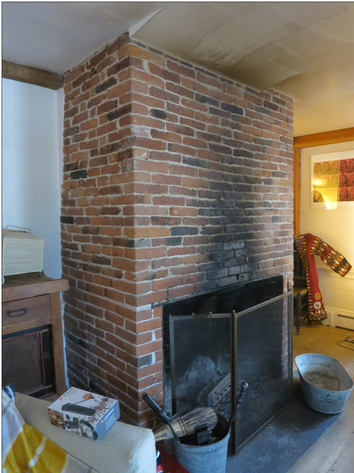
First floor fireplace and chimney.
