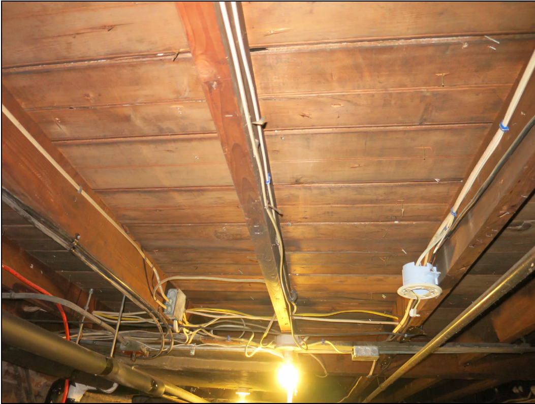
First floor beams and flooring from basement.
