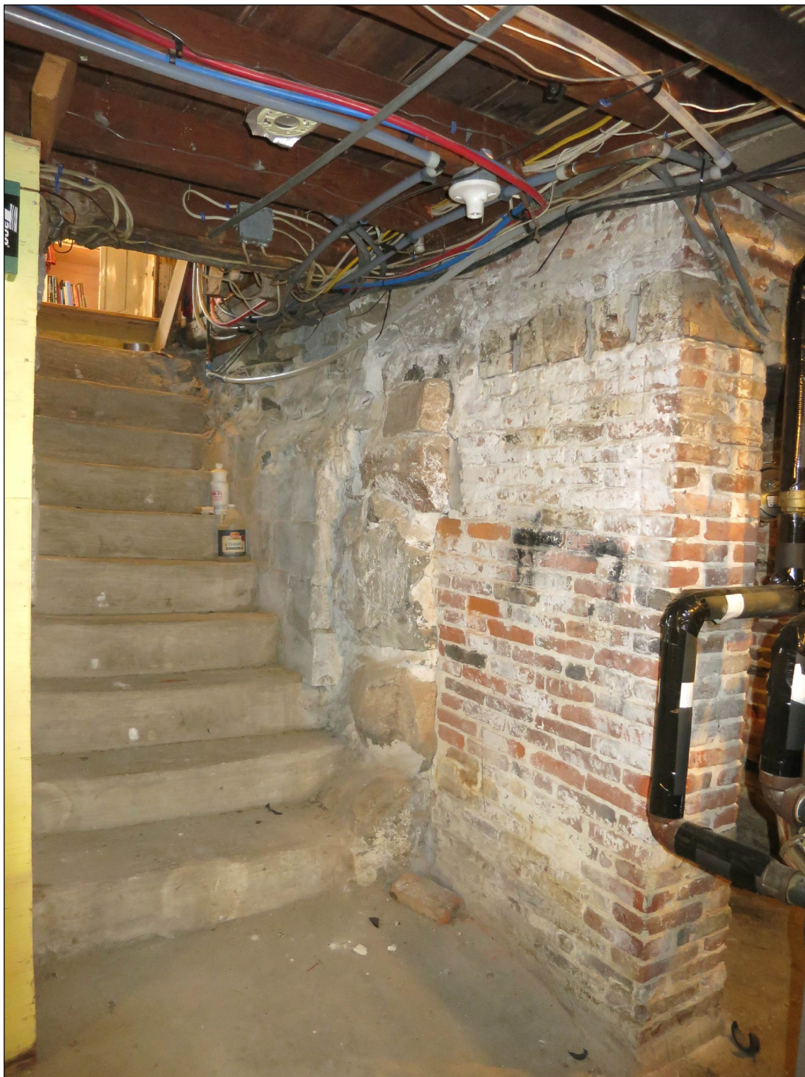
Basement stairs to lean-to. Chimney base on right.
