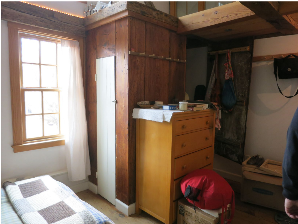
Box stair in corner of SE room
