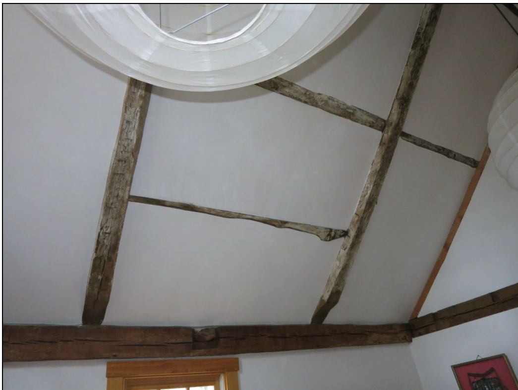
Second floor, NE room, showing roof framing.
